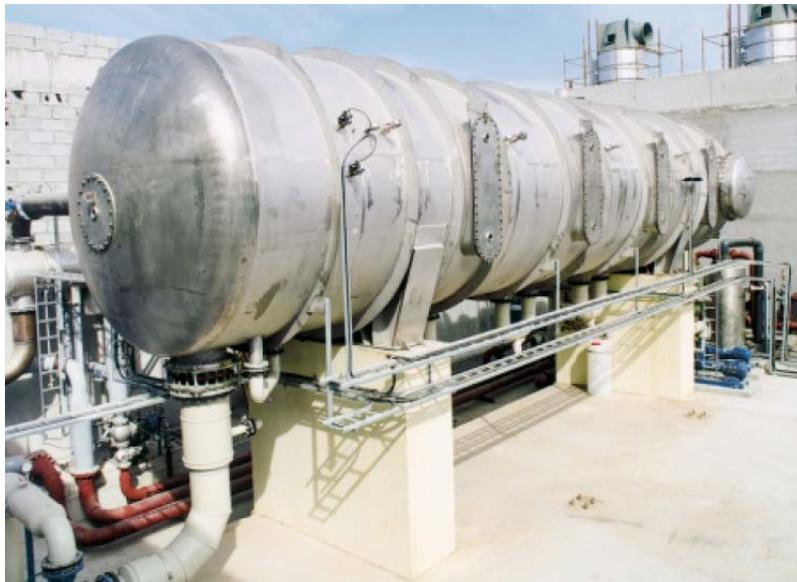
**Fig. 6** Alfa-Laval MED desalination unit using plate type heat exchangers.
