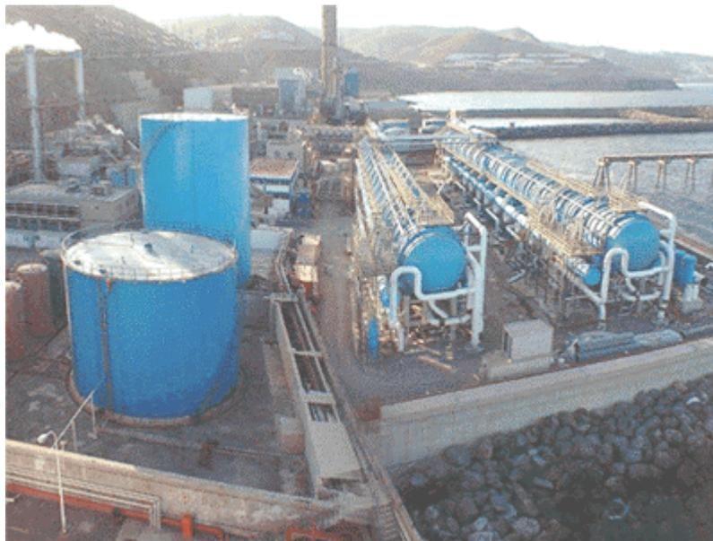
**Fig. 2** A 2-unit MED plant built by IDE Technologies with total capacity of 35,000 m<sup>3</sup>/day (<http://www.ide-tech.com/code/what.html>).
