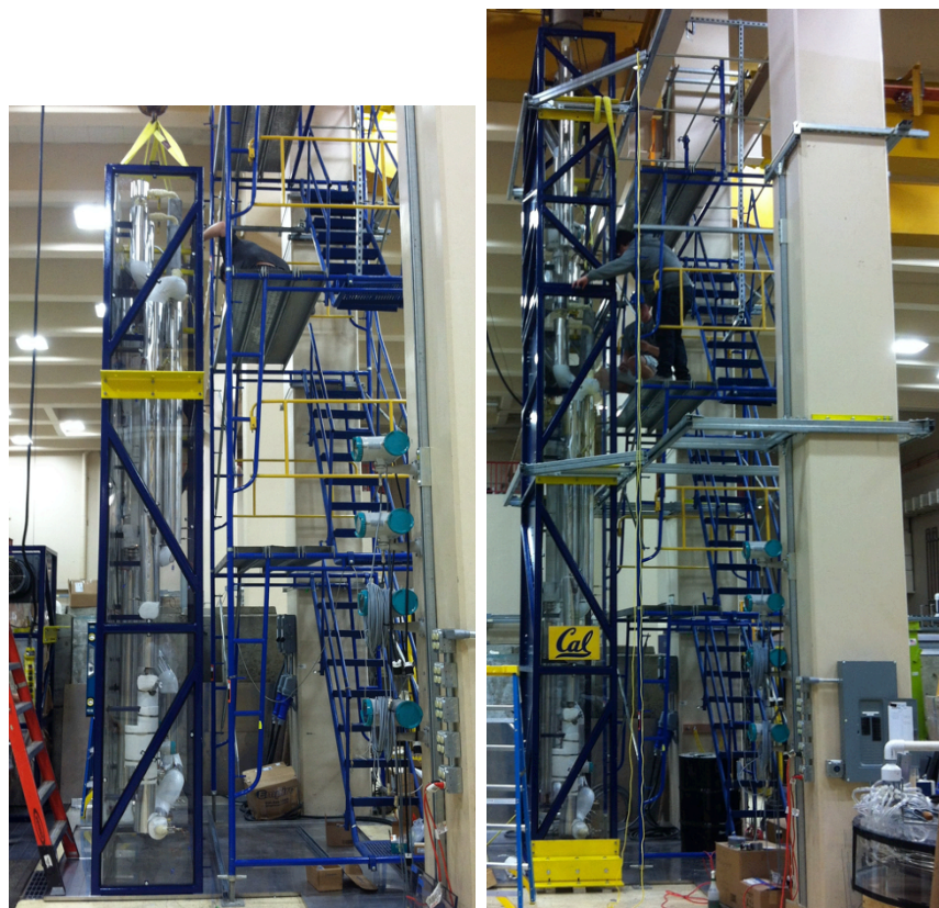
Figure 3-18. CIET 1.0 lower frame assembly (left) and upper frame assembly (right) being set in place, June 2014.
