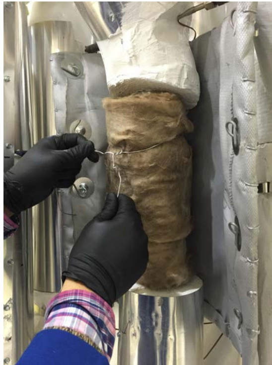
Figure 4.12. Installation of flexible fiberglass insulation underneath thin, removable insulating pads.
