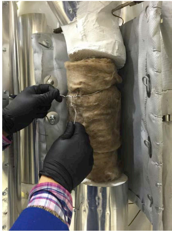
Figure 59. Installation of flexible fiberglass insulation underneath the removable insulating pads.
